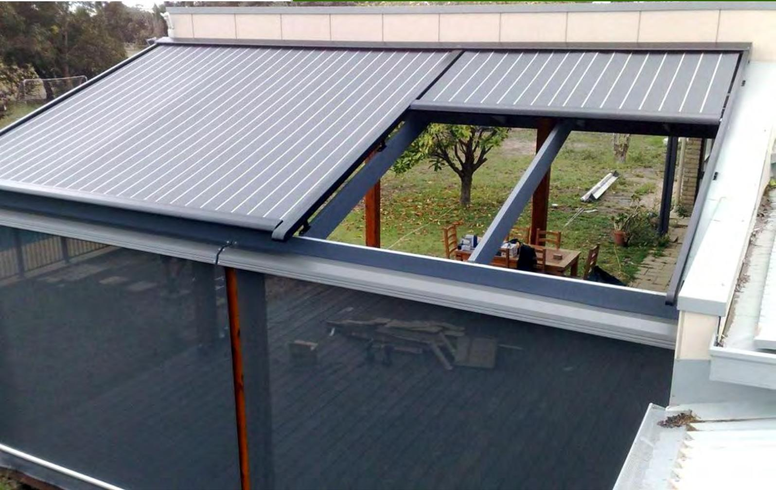
Harol Conservatory awnings when rolled up the fabric is completely inside the VZ box, protected against any effects of the weather outside. The VZ is fixed to the guide rails, which are fastened to the conservatory frame by means of fastening supports.
